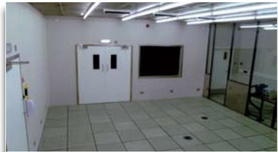
Bassaire constructed the full unidirectional room with over 500 air changes per hour; Bassaire also manufactured the full stainless steel LAF ceiling.
