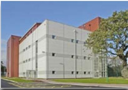
The new laboratory building (referred to as Unit 11 Quality Control (QC) Laboratories) comprises of a four-floor building in which the ground floor of the building houses the Microbiology Laboratories and the first floor will house the Analytical Laboratories. The second floor has been left as an empty open plan area for future use and the third floor houses a plant area.
